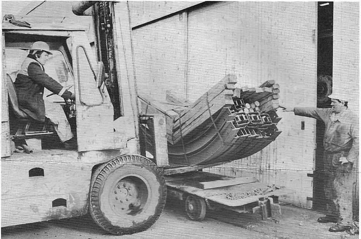
A package of girders ready to go underground
