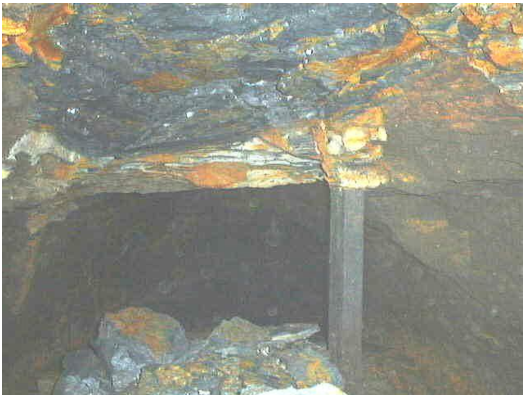
Tunnels in the underground workings of Alice Pit, Begg Colliery
