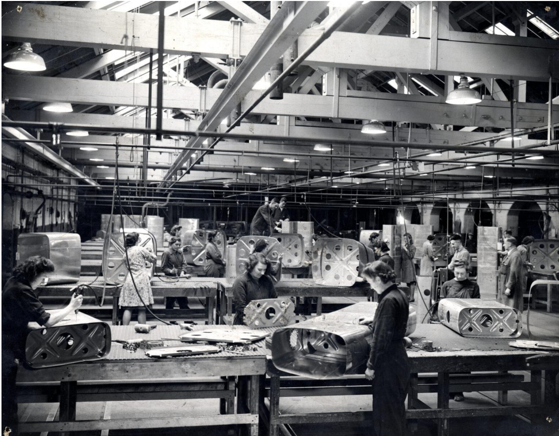
Workers at Michael Nairn and Co. Ltd. Making fuel tanks for Halifax bombers. Both Barry's and Nairn's manufactured goods for the war effort in WWI and WWII.
